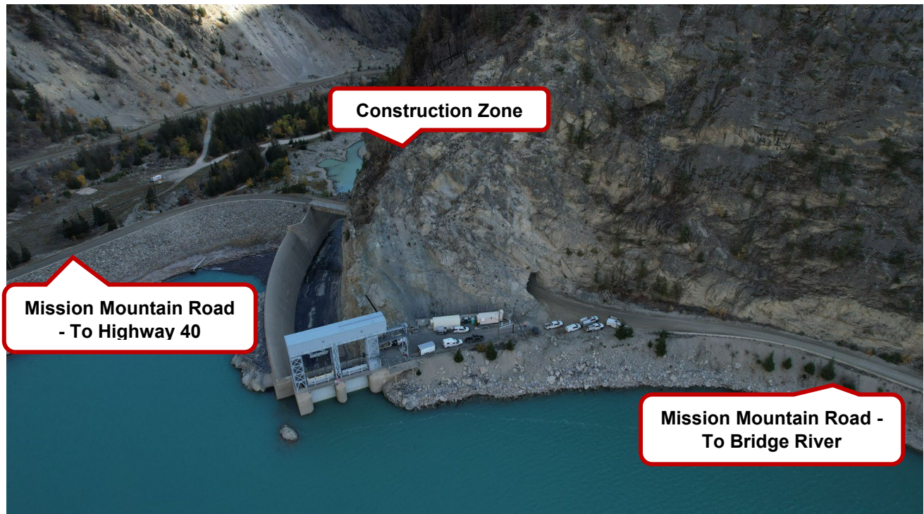
Above: The work zone on Mission Mountain Road to Bridge River, Squamish-Lillooet.
