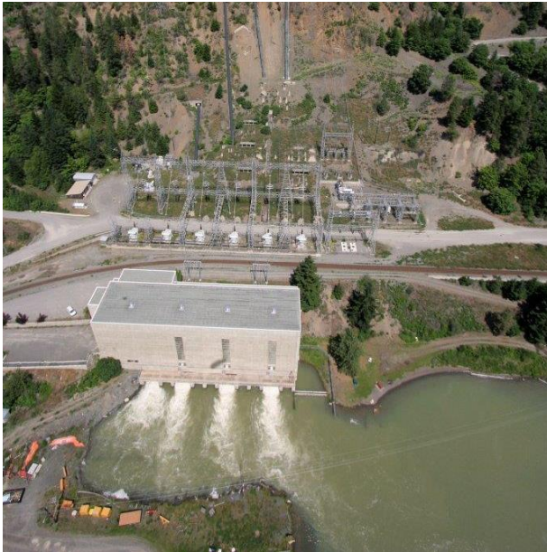
Aerial view of Bridge River Generating Station – Unit 1
