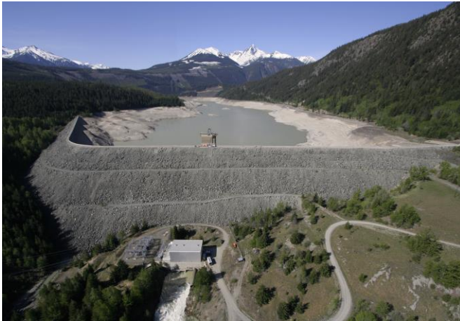
LaJoie Dam with Downton Reservoir in the background and a 25 MW powerhouse in the foreground
