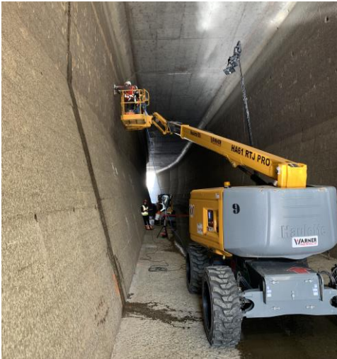
Crews extracting coring samples in Seton Canal, spring 2022
