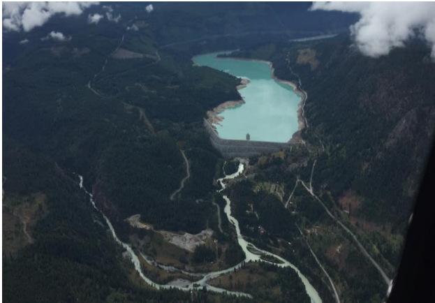
Aerial view of LaJoie Dam with Downtown Reservoir behind it
