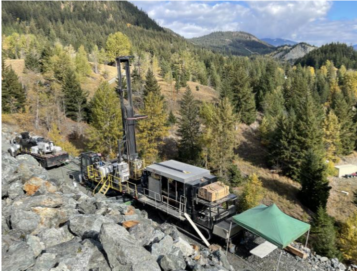
Drilling rig on La Joie Dam during site investigations (September 2023)
