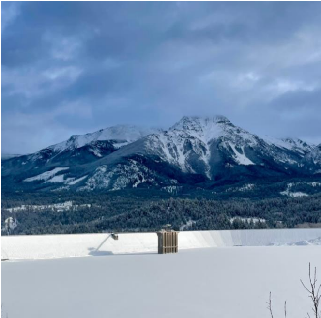
Truax mountain overlooking a snow covered La Joie Dam and the intake tower with Downton Reservoir in the foreground
