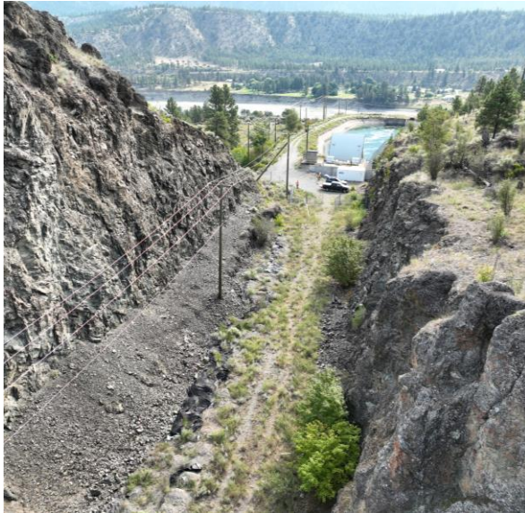
Drone photo of the rock slope along the bypass route with the Seton forebay in the background (July 2023)
