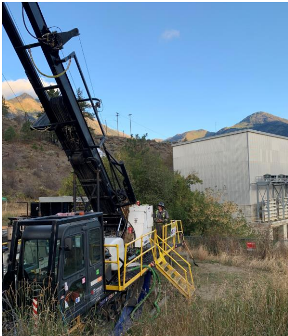
Crews drilling near the outlet of the bypass (Sept. 2023)
