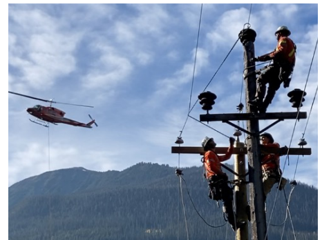
Malm with 2 colleagues working on pole replacements alongside a helicopter just outside Bralorne.
