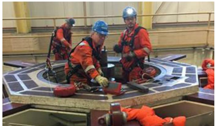
Crews preparing for Unit 5 upper bracket removal on the Bridge 2 Units 5 and 6 upgrade project. Similar work will take place as part of the Bridge 1 upgrade.
