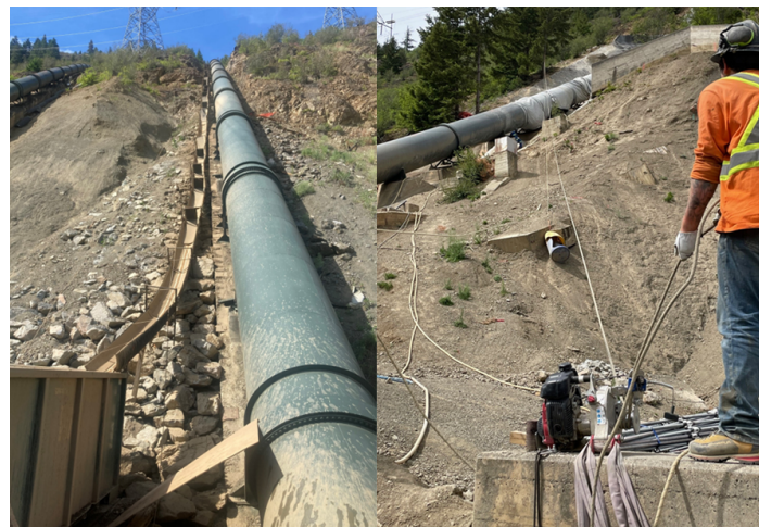
An innovative flume system designed to remove debris from the slope (left) and a worker operates a tight light handling system to ergonomically transport materials on the slope (right).
