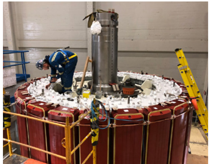
A crew member touches up paint on a rotor at BR2.
