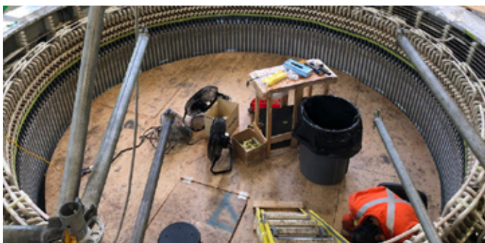
Crews have been busy with the pre-assembly work for units 7 and 8 at BR2.
