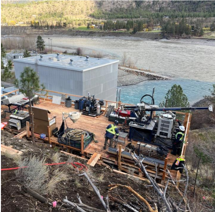
Crews drilling at the bypass tunnel portal (Nov. 2024)
