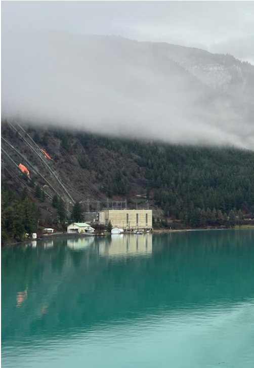
Bridge River Generating Station – Unit 1
