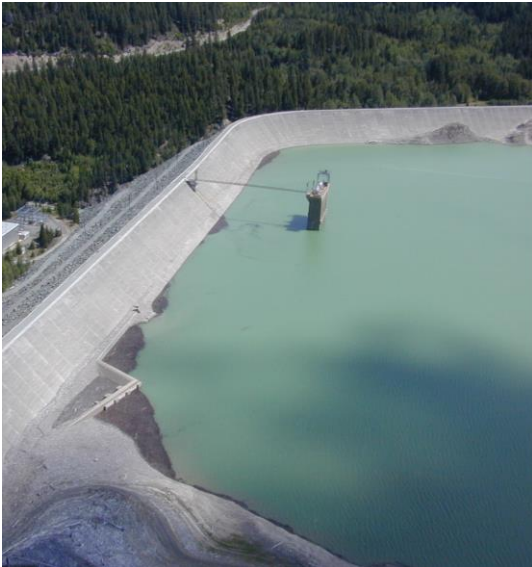
La Joie Dam and the intake tower standing in Downton Reservoir
