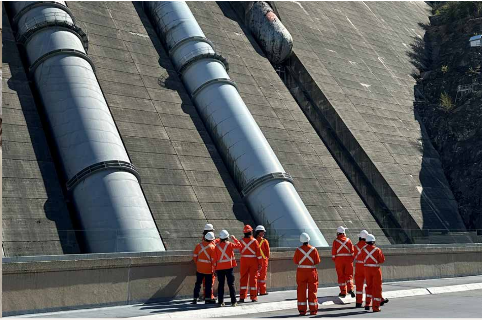
Space for new penstock
