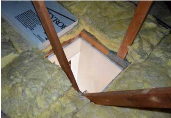
Attic access hatch with insulated gypsum cover
