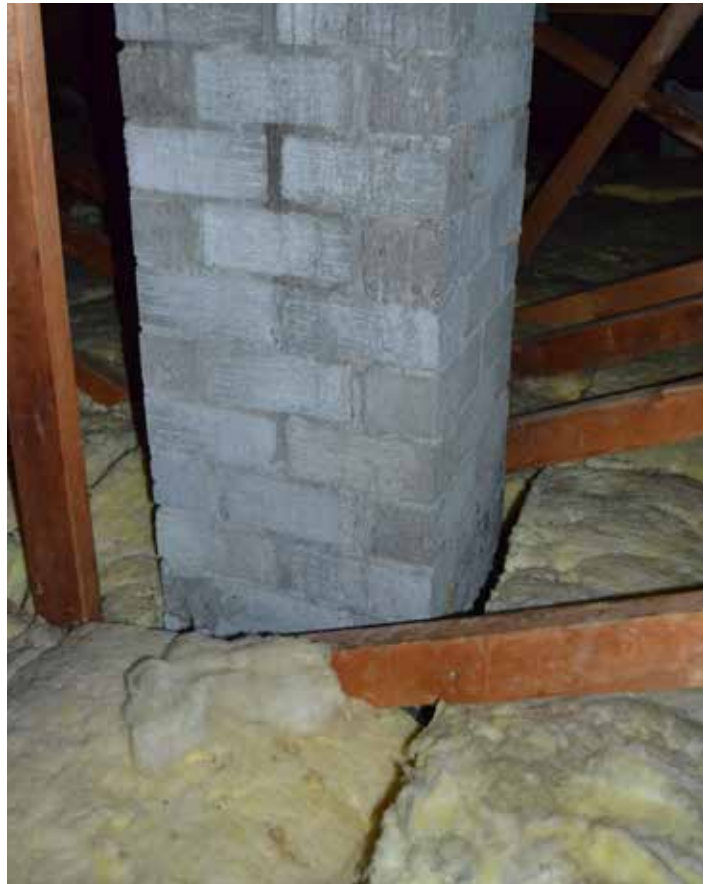
Three-inch gap around chimney
