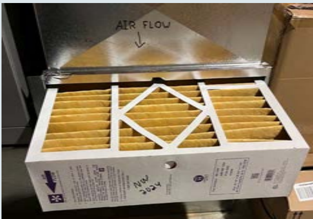
Figure 5 Example of Larger Filter
