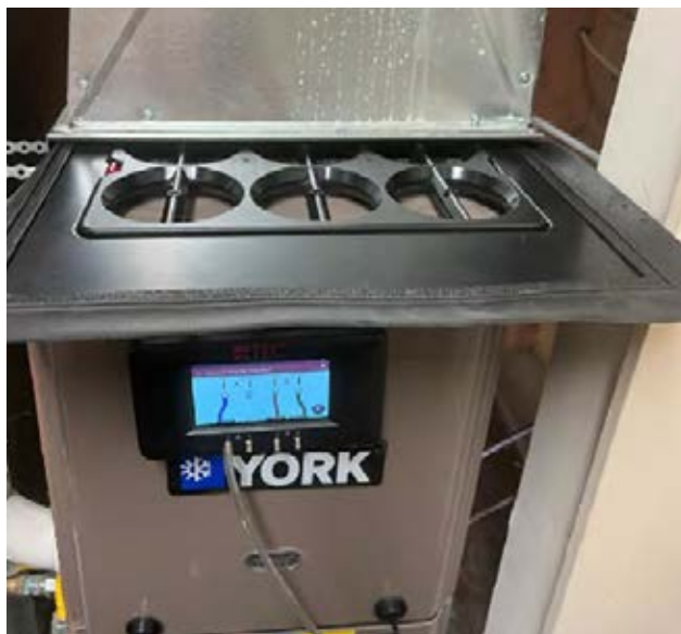
Figure 4 Testing Existing Ductwork Capacity - Air Flow (Flow Grid)
