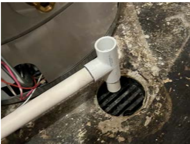
Figure 18 Condensate Management for Lateral Drainage Pipe
