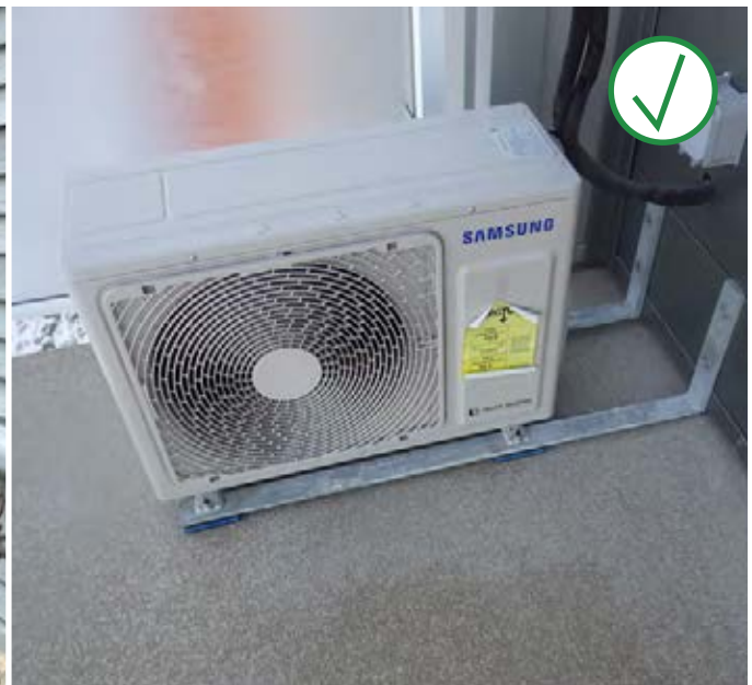
Figure 11 Example of Installation with Inadequate Clearance (left) and Adequate Clearance (right)
