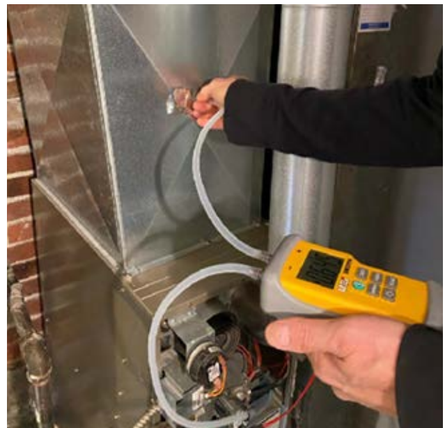
Figure 3 Testing Existing Ductwork Capacity - Static Pressure Test (Supply Only Location)
