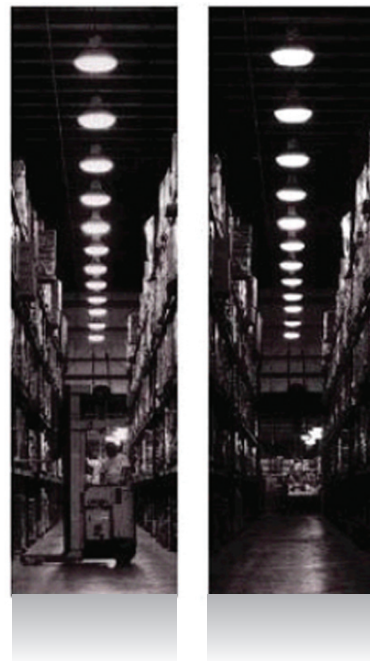
Full Power (Left) and Dimmed (Right) High Bay Lighting
