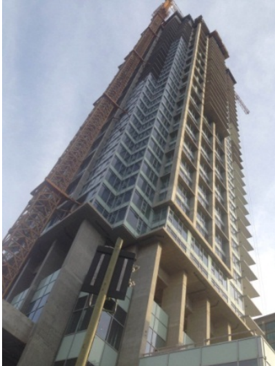
Figure 3.8: A common form for a residential tower in BC with many thermal bridges at interface details
