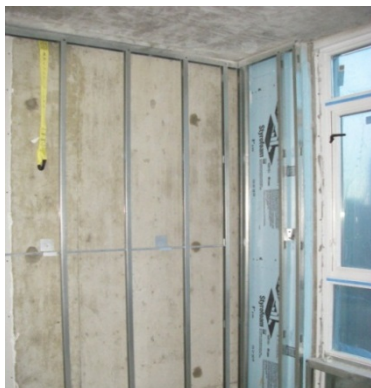
Figure 3.9: A concrete shear wall bypasses the thermal insulation (seen from the interior). The blue material is insulation, is on both sides of the concrete wall. The concrete wall is part of the suite separation.
