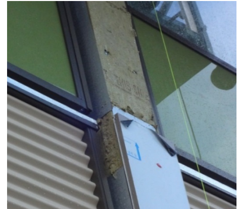
Figure 3.5: An example of thermal bridging at the interface between assemblies. This is NOT captured by wall schedules but reduces the insulation effectiveness
