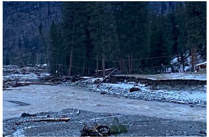
Flooding and BC Hydro infrastructure damage in Merritt, B.C., November 2022.
