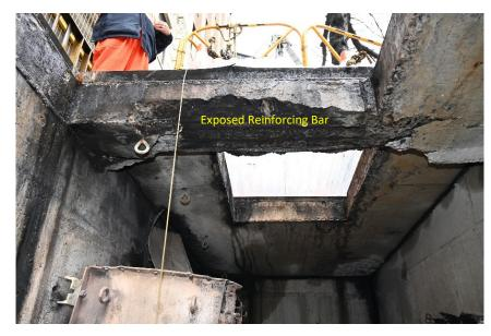
Figure 16: Vault structural damage.
