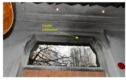
Figure 10: JJBean interior smoke extension dominant through south end of window.
