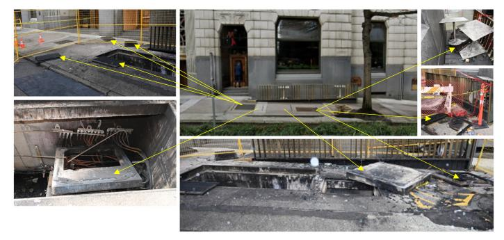
Figure 4: Photo array showing vault debris displacement.
