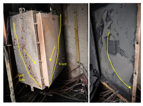
Figure 24: Front-left side of CLF (left); inside of cabinet door (right).
