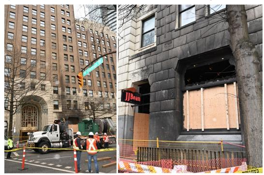
Figure 8: Marine Building façade damage.
