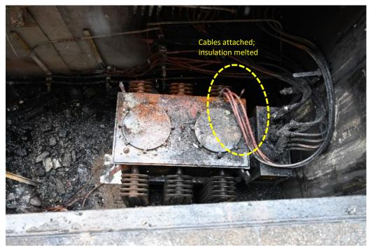
The transformer had three insulated supply cables terminating on the front face of the housing (north side) connecting to the fuse cabinet. Four sets of four insulated distribution cables exited the transformer at the back
