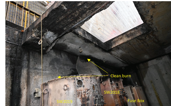
Figure 14: Ceiling on the west side at the north end of V73.
