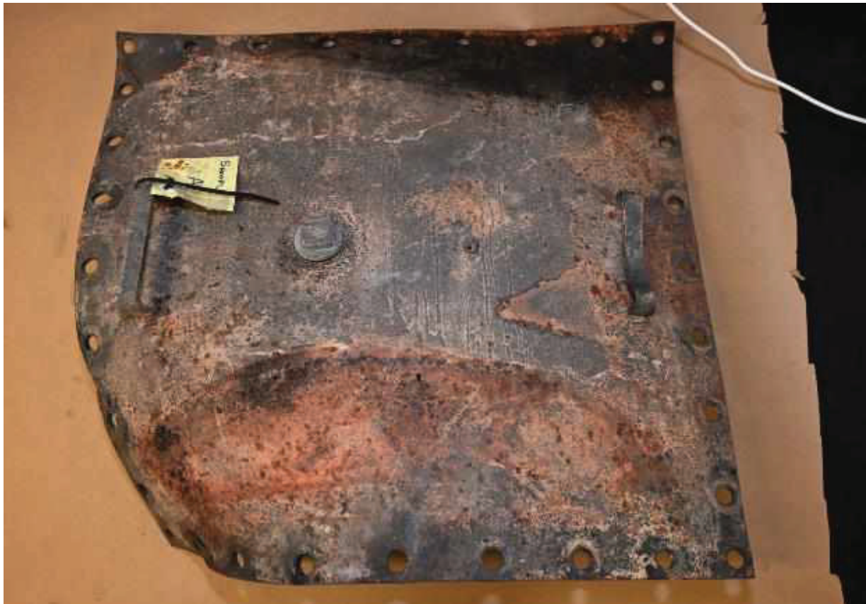
Figure 4. Bent lid from switch 2019
