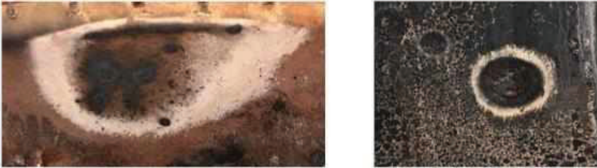
Figure 5. Close up of white rings on inside of the switch 2019 tank
