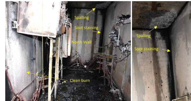
Figure 13: V73 north wall.
