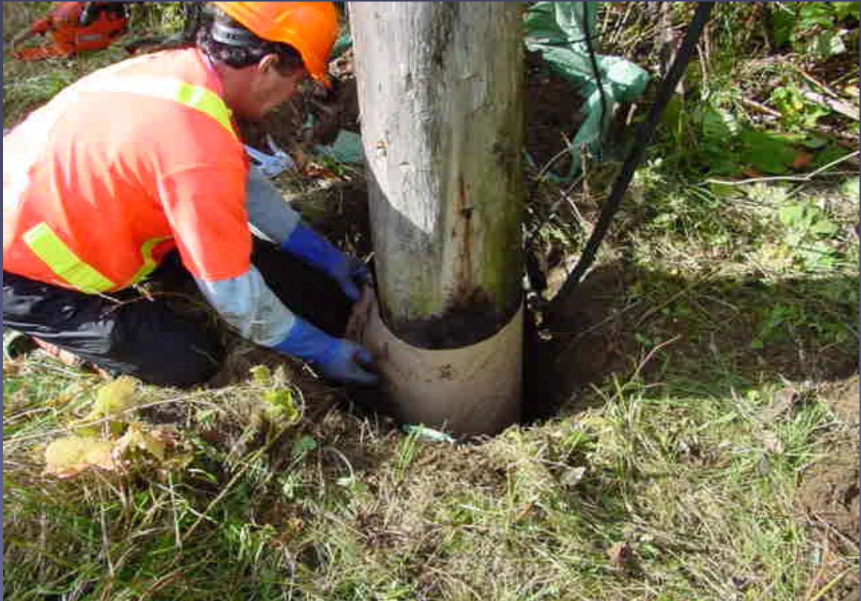
Installing a full bandage
