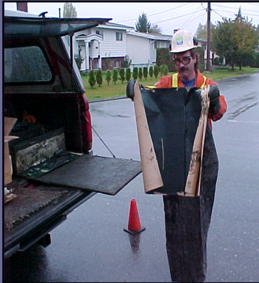
Field-Made Pole Bandage
