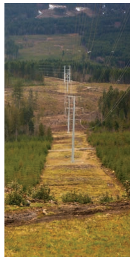
One of our transmission line corridors.
