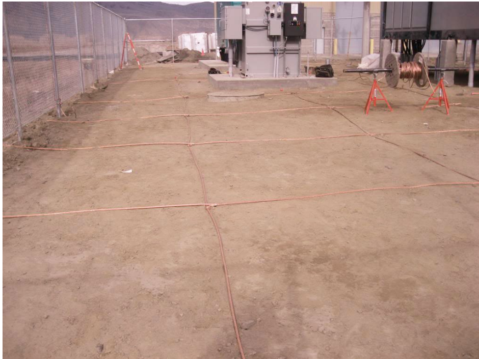
Copper ground grid before being covered
