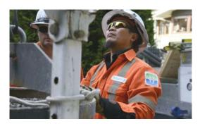
3. Next, the Category 5 worker isolates the customer from BC Hydro's power system. This is done by opening a switch or other device to create a positive isolation point.
