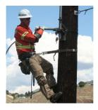
3. The BC Hydro Category 5 worker removes the lock and tag and then closes the switch or device to reconnect the customer to the power system. The worker then advises the customer that the line or equipment is energized.
