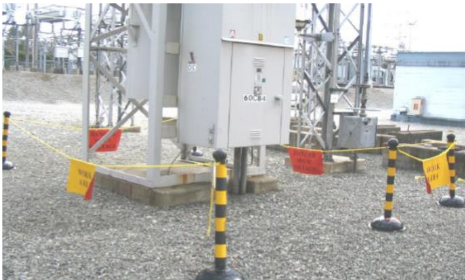
Figure 2. Work area barriers defining safe work area
