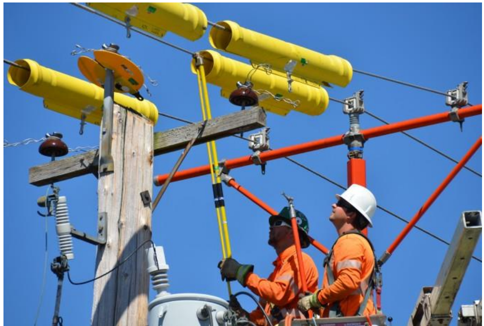
Figure 4. Use of live-line tools
