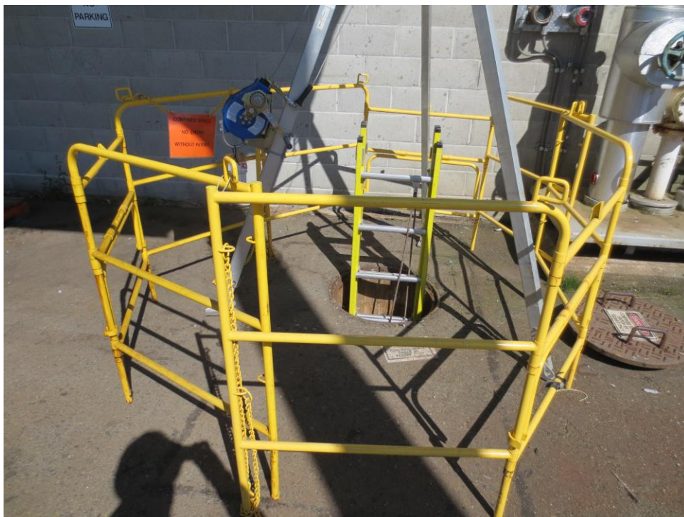
Figure 3. Work area barriers defining a hazard zone
