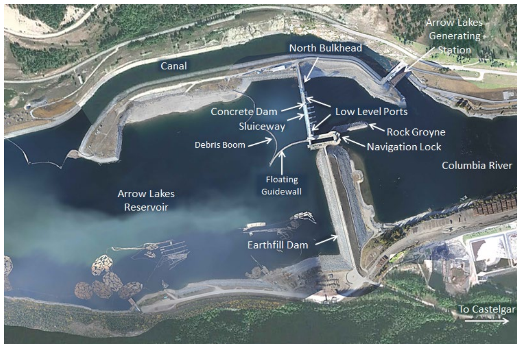
Figure 4: Hugh Keenleyside Dam Site Layout.
