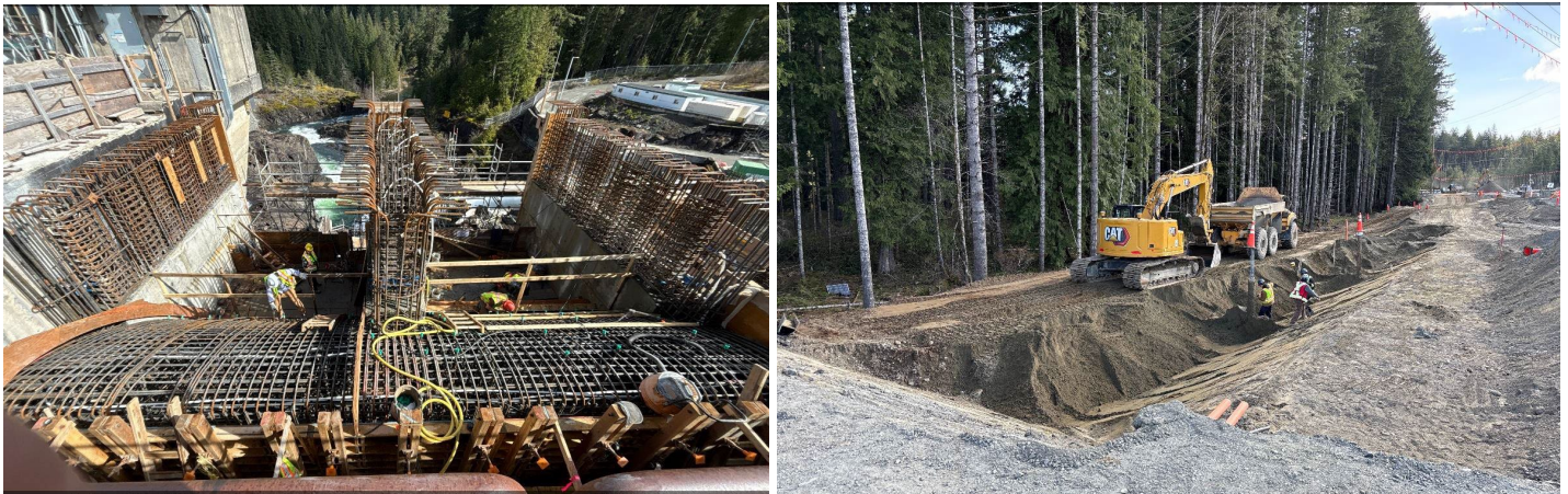
Figure 8 John Hart Dam Seismic Upgrade Project. Left: Construction of ogee spillway crest; Right: Excavation of south bank drain.
