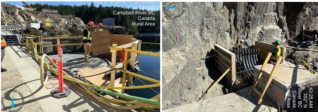
Figure 7 Ladore Spillway Seismic Upgrade Project. Left: Containment setup for post-tensioned anchor drilling; Right: Electrical ducting installation.
