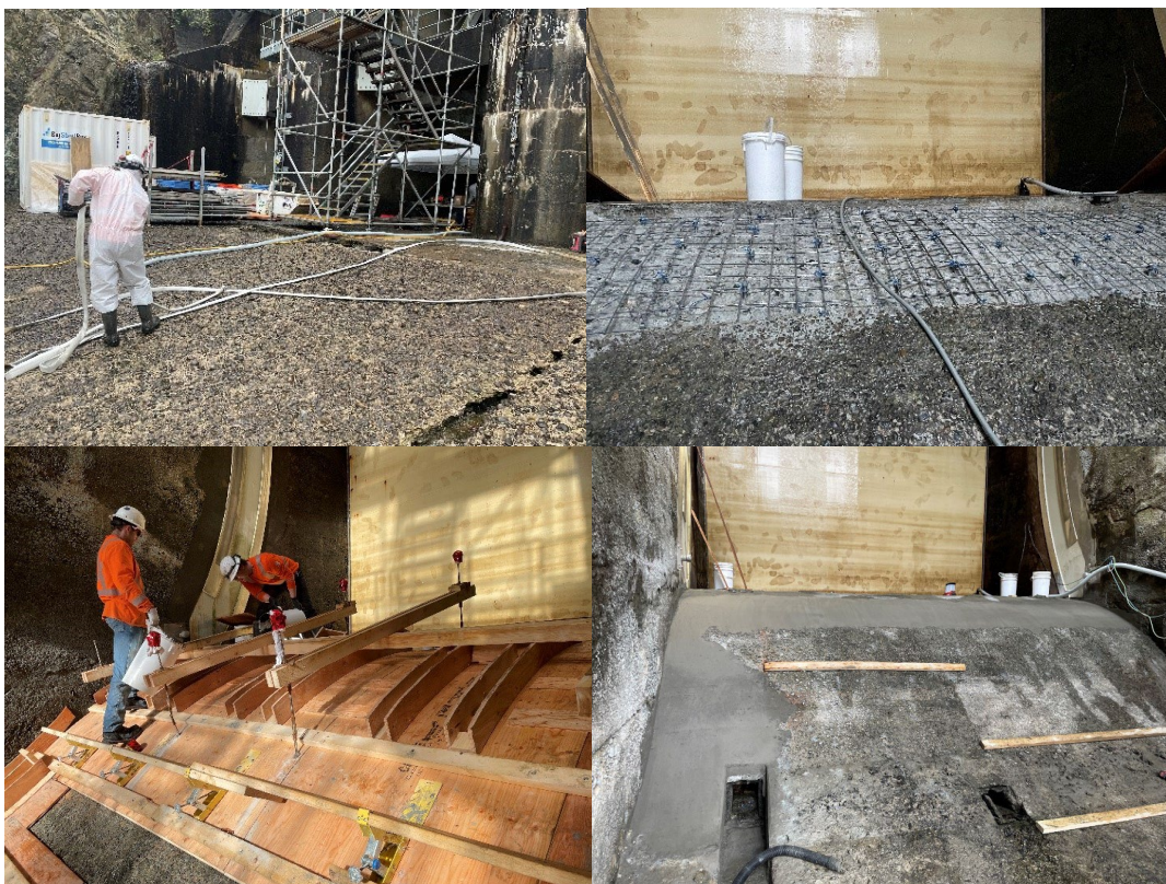
Figure 4 Stave Falls Spillway Bay 2 Concrete Repairs. Top Left: Scaffolding installation for access and egress into spillway bay 2. Top right: Installation of welded wire mesh following removal of deteriorated concrete. Bottom left: Curved form work in preparation of concrete placement. Bottom right: Concrete placement.
