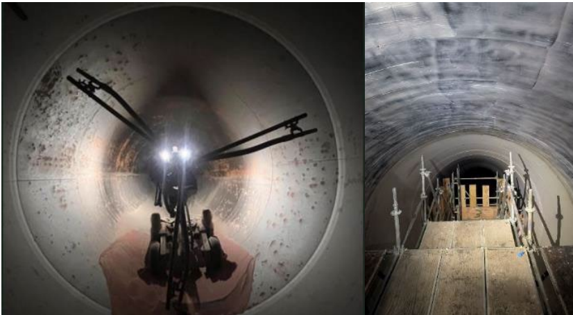
Figure 11 Left: Penstock recoating robot. Right: Carbon fiber reinforced polymer sleeve.
