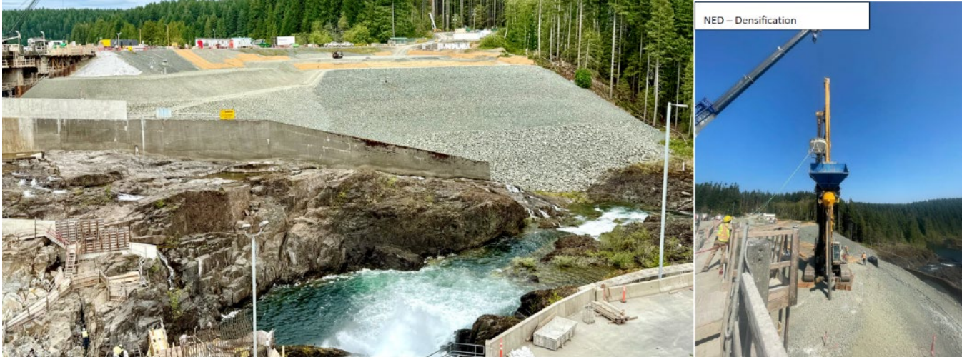
Figure 9 Downstream side of the John Hart North Earthfill Dam and the downstream berm and ground improvements
