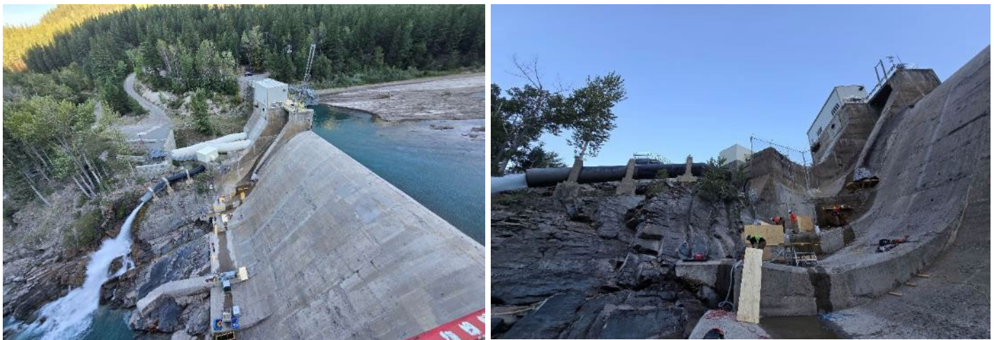
Figure 6 Aberfeldie spillway repairs. Bottom left: Overview of the spillway overflow channel and work area. Bottom right: Construction Services team preparing for formwork installation at a repair location.
