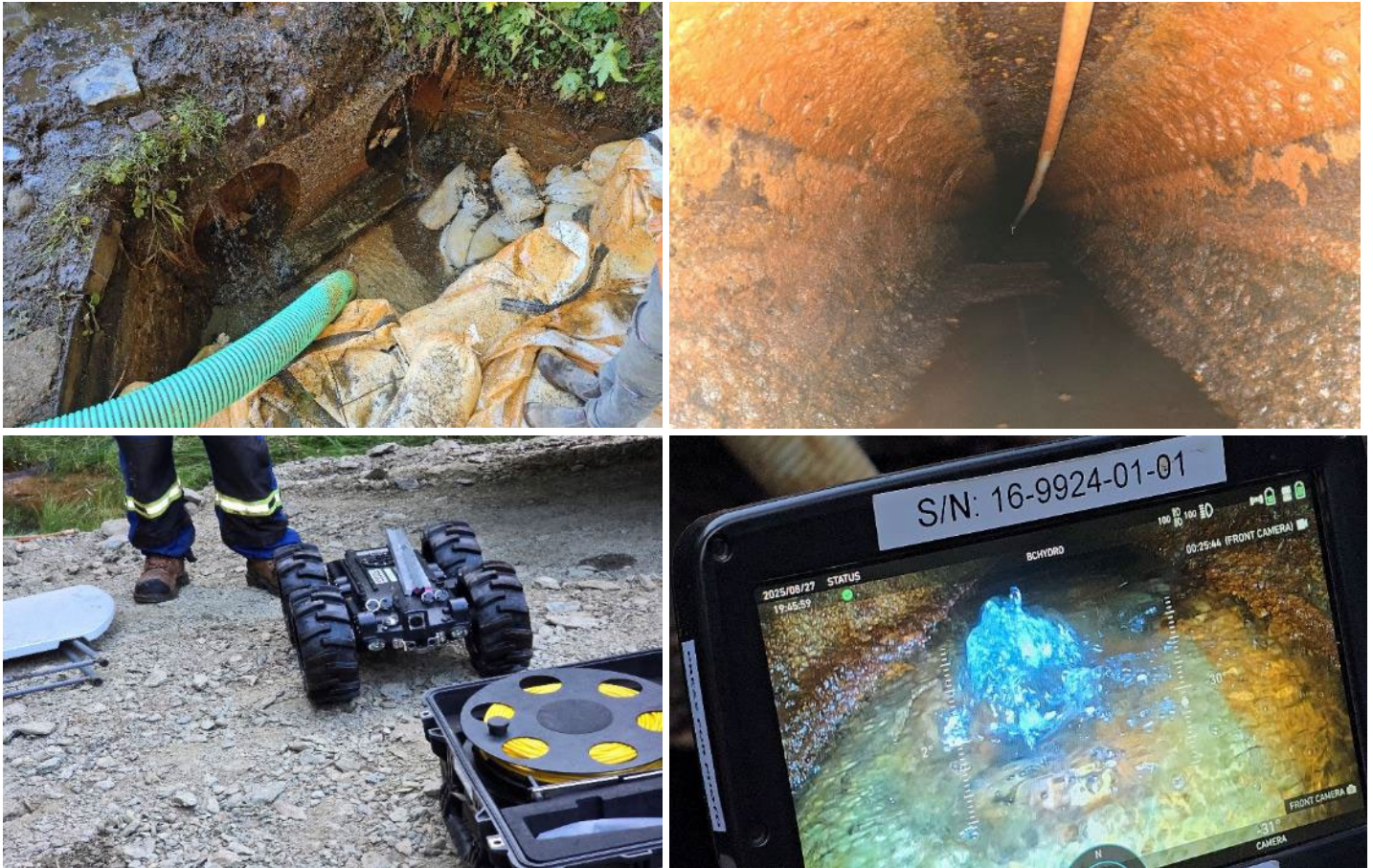
Figure 4 Seepage into the left Low Level Outlet pipe through holes in the rivetted steel pipe.
