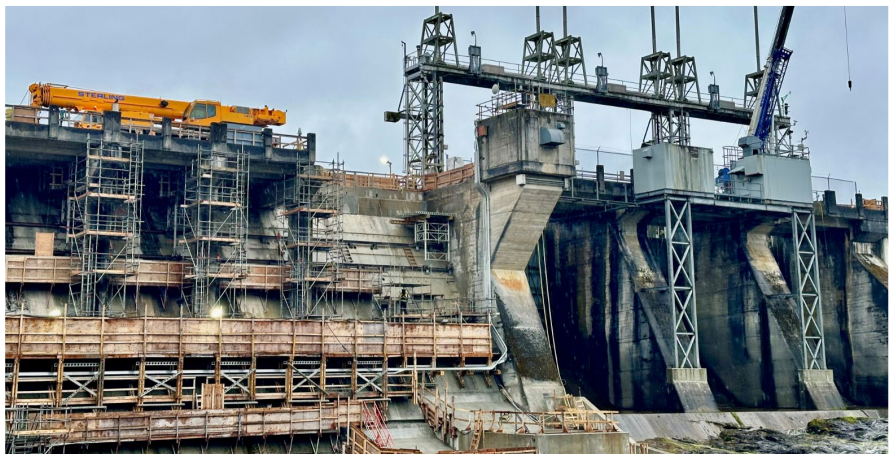
Figure 9 Construction on the John Hart Dam Seismic Upgrade Project. Top: April 15 view of the Middle Earthfill Dam on the left and the North Earthfill Dam on the right. Middle: April 15 view of the work on the berm to stabilize the Intake Dam. The berm will be built up to the old dam. Bottom: April 8 view of the Concrete Main Dam, showing the removed section of roadway deck adjacent to the spillway.
