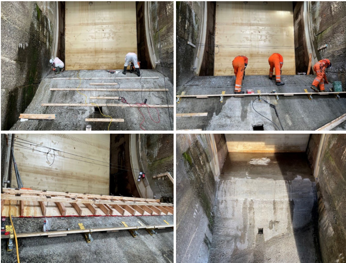
Figure 6 Stave Fall Spillway Bay 1 Concrete Repairs. Top left: Removal of deteriorated concrete downstream of the of the sill beam. Top Right: Cleaning, surface preparation and reinforcement installation. Bottom left: Curved formwork installation in preparation for concrete placement. Bottom right: Completed concrete repair.
