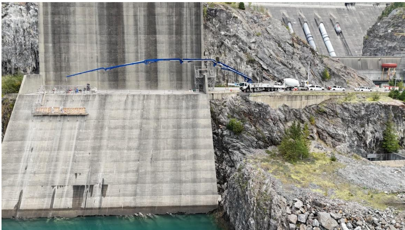
Figure 4 Concrete repairs underway on the downstream slope section of the spillway at Revelstoke Dam, directly above the plunge pool.
