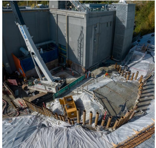
Figure 8 Pile shoring nearing completion on the left abutment of Ruskin Dam.
