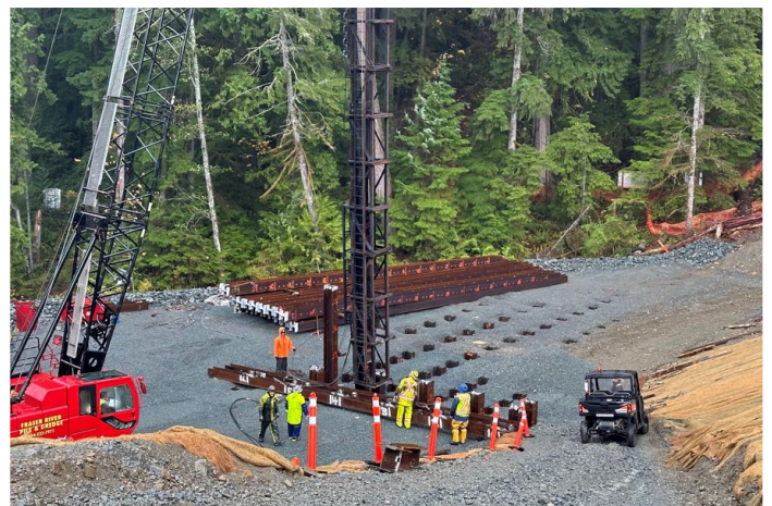
Figure 7 Construction on the John Hart Dam Seismic Upgrade Project. Top: Main Concrete Main Dam. Middle: H-Pile installation on the toe of the Middle Earthfill Dam. Bottom: Close-up of H-pile installation.
