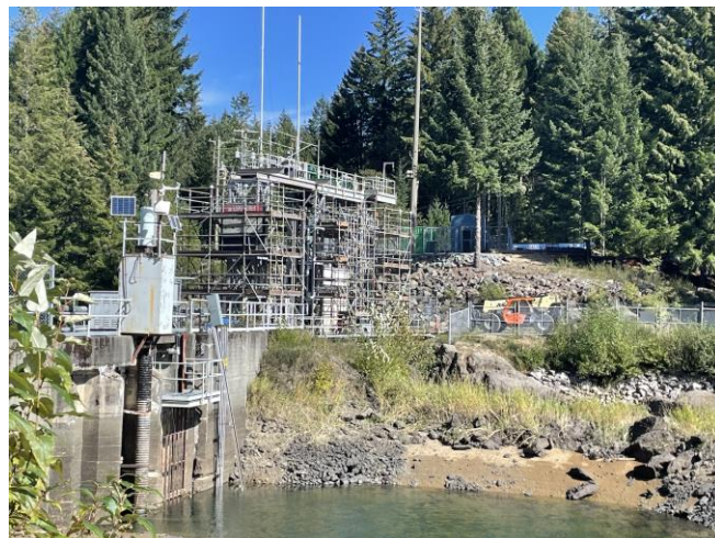
Figure 6 Construction scaffolding surrounds the spillway gate hoist structure at the Comox Dam in September.
