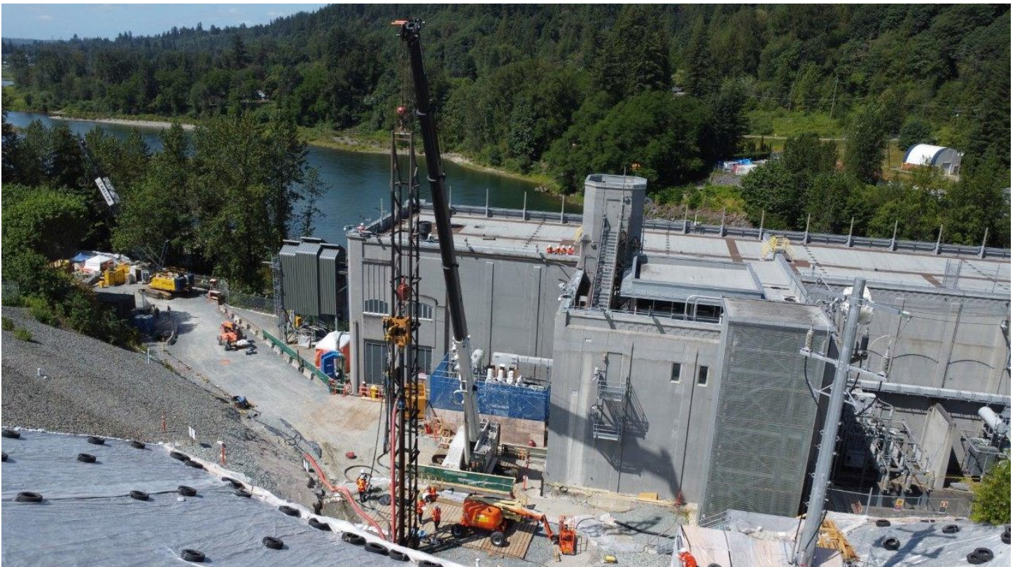
Figure 8 Left abutment of Ruskin Dam adjacent to the powerhouse. Pile driving is underway to construct shoring walls for excavation of erodible sub-surface clays. Polyethylene sheets that are being used to protect the slope from water infiltration during heavy precipitation events are visible in the foreground.
