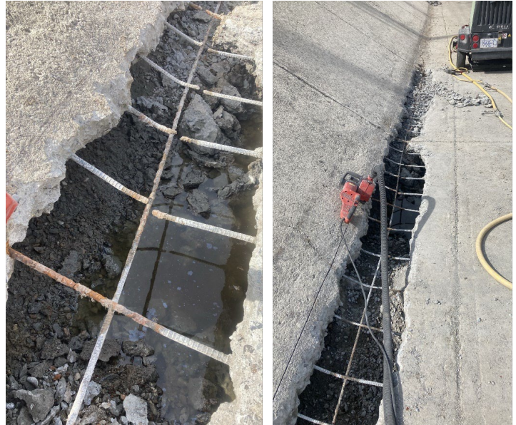
Figure 9 Water-filled void found under the Seton Canal during concrete remediation works.
