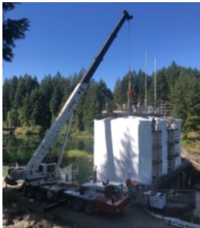
Figure 6 Spillway at Comox Dam in early July. Hoarding is being installed in preparation for work to upgrade the spillway gates.
