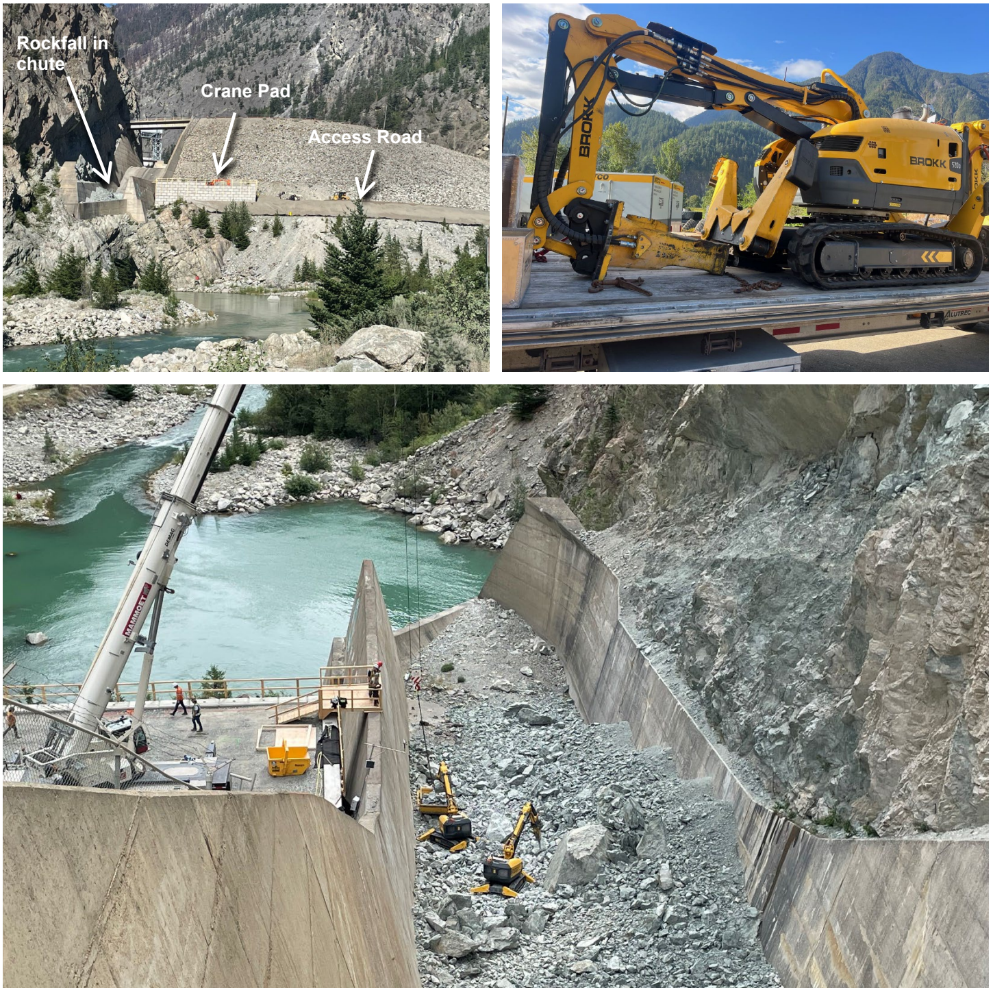
Figure 3 Progress in the work to remove rockfall from the Terzaghi Dam spillway chute. Top left: the access road and crane pad, shown near completion in early July. Top right: one of the remotely controlled demolition and excavation units being readied for mobilization to site. Bottom: excavation underway as of July 25, 2024. The excavator operators can be seen on the wooden platform on the left side of the spillway chute.
