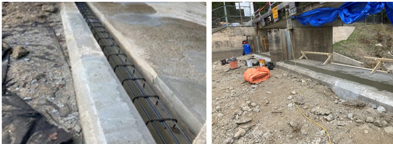
Figure 4 Repairs of stoplog sill at Whatshan Dam. At left: Completed removal of deteriorated concrete and newly installed reinforcement. At right: Completed concrete placement.
