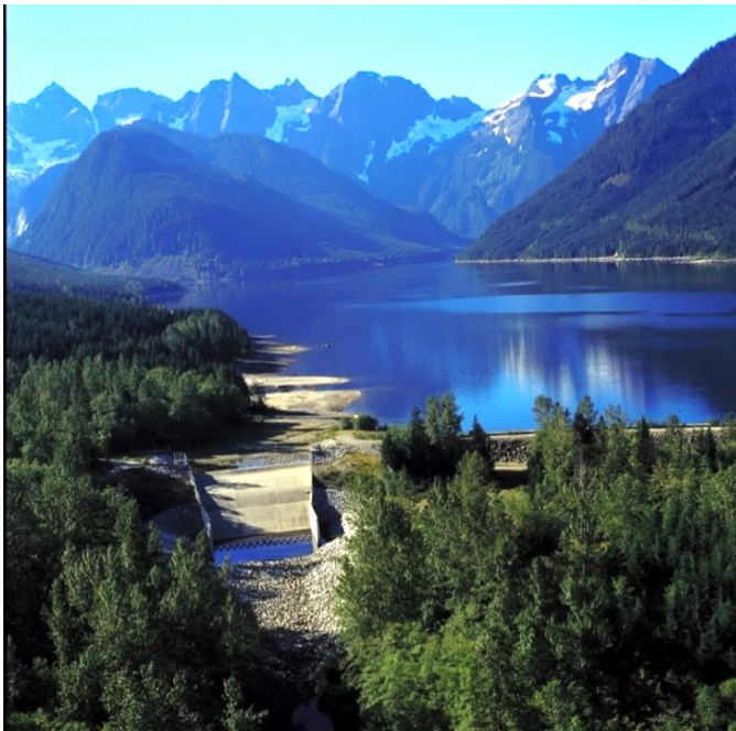
Jones Lake and Wahleach Spillway
