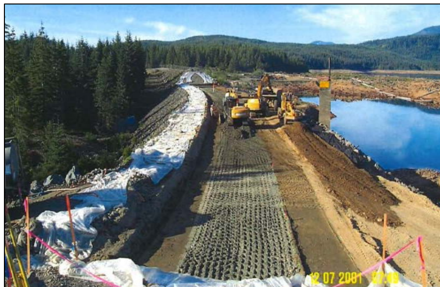
Saddle Dam 1: Reconstruction of dam in 2001
