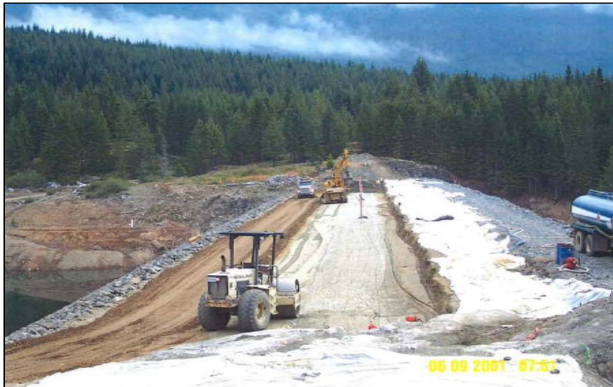
Main Dam: Compacting new fill placement (Crest View)
