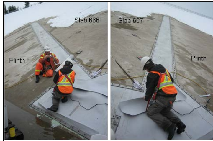
(Left) 2009 CARPI geomembrane on Slabs 579 and 578; (Right) 2009 CARPI repair on Slabs 666 and 667 on south forebay (left, upstream; right, downstream sides of Chevron)
