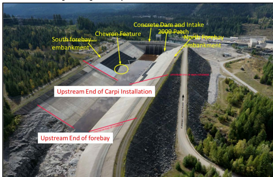
2014 Completion of the Forebay CARPI geomembrane and drainage system
