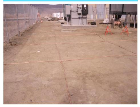
Copper ground grid before being covered
