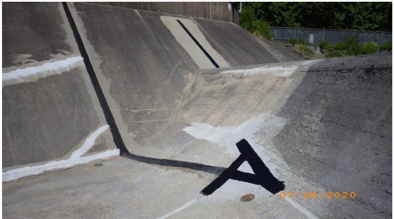
Figure 4 Alouette spillway concrete joint repairs.
