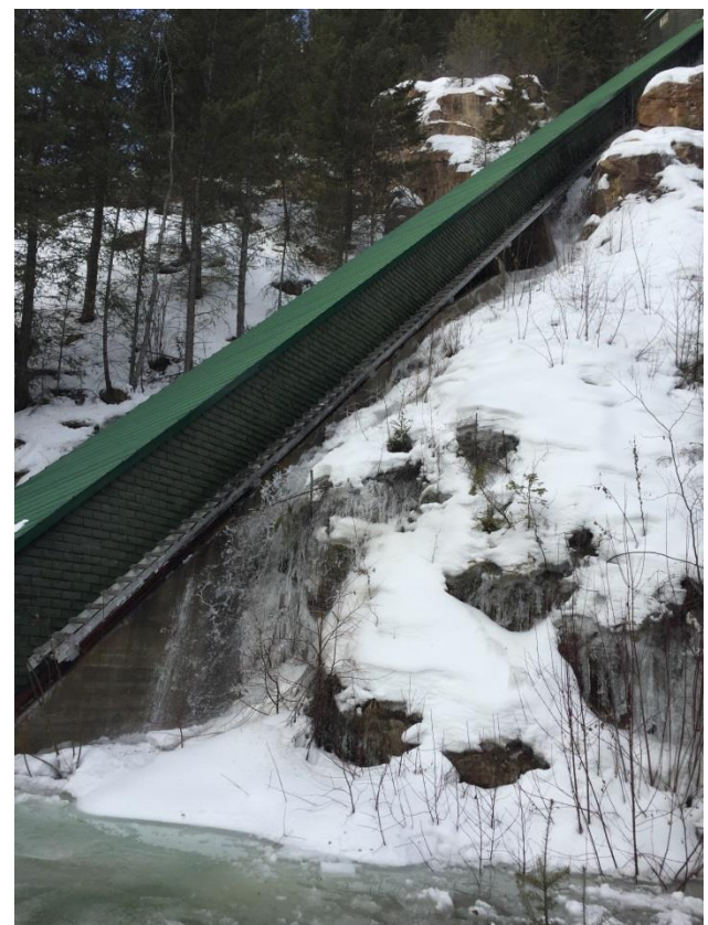
Figure 6 Water cascading down the slope adjacent to Penstock 01/02 along a channel eroded through the soil overburden.
