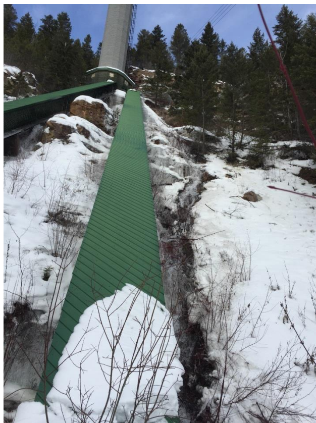
Figure 6 Water cascading down the slope adjacent to Penstock 01/02 along a channel eroded through the soil overburden.
