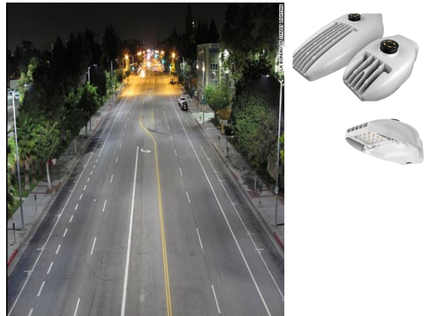
New LED Street Lights
