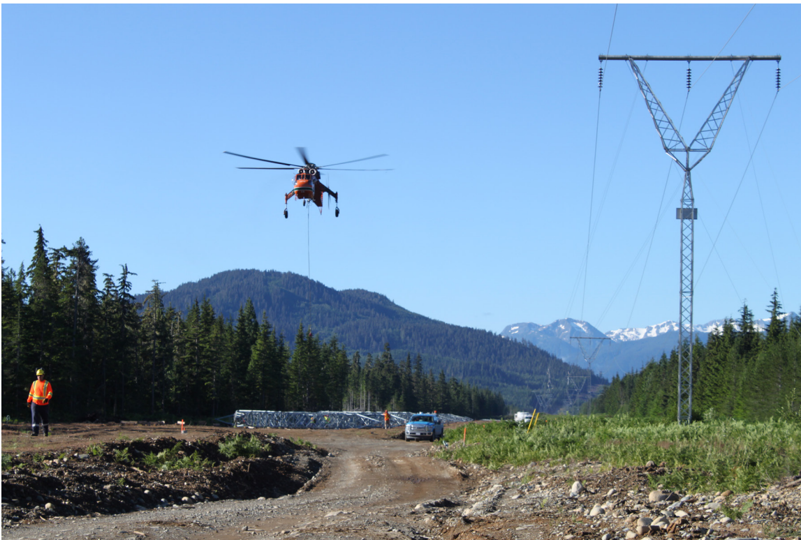
Transmission tower installation with helicopter assistance.
