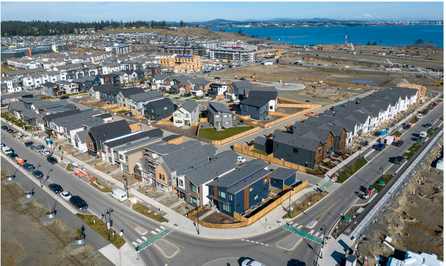
New residential construction in Colwood.
