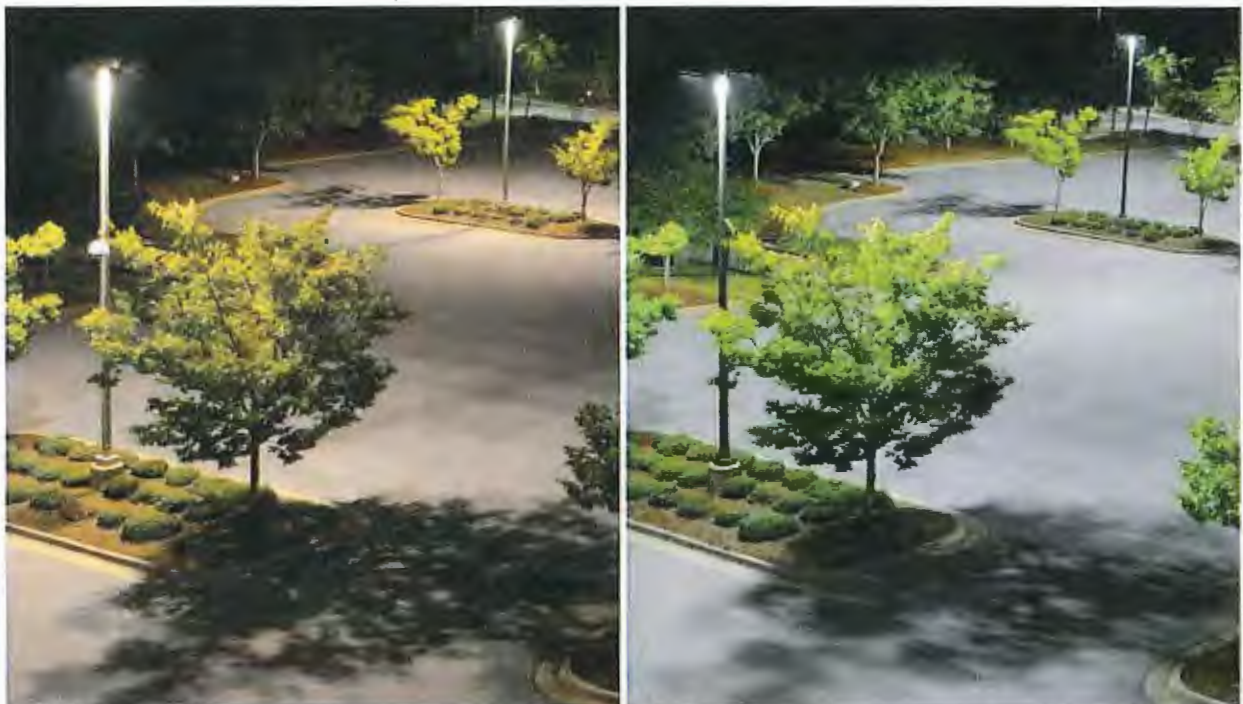
High pressure sodium streetlights (left) that have been replaced with light emitting diodes (right).
