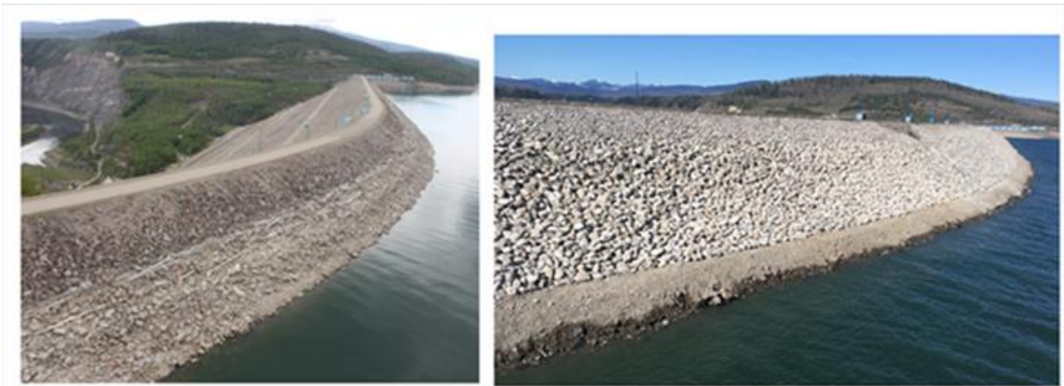
4 Figure 2 Before and after Riprap Placement
