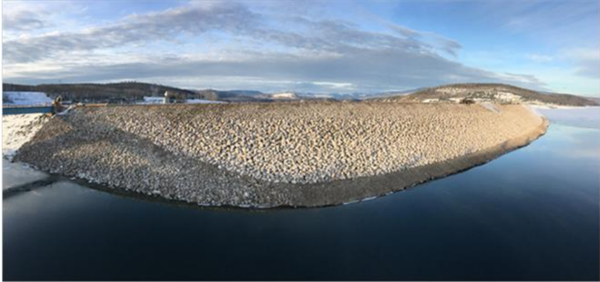
2 Figure 1 WAC Bennett Dam Riprap Project 3 Completion
