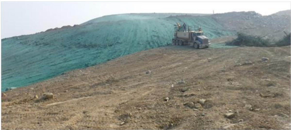
Figure 5 Hydro-seeding after Filling and Smoothing of Topsoil
