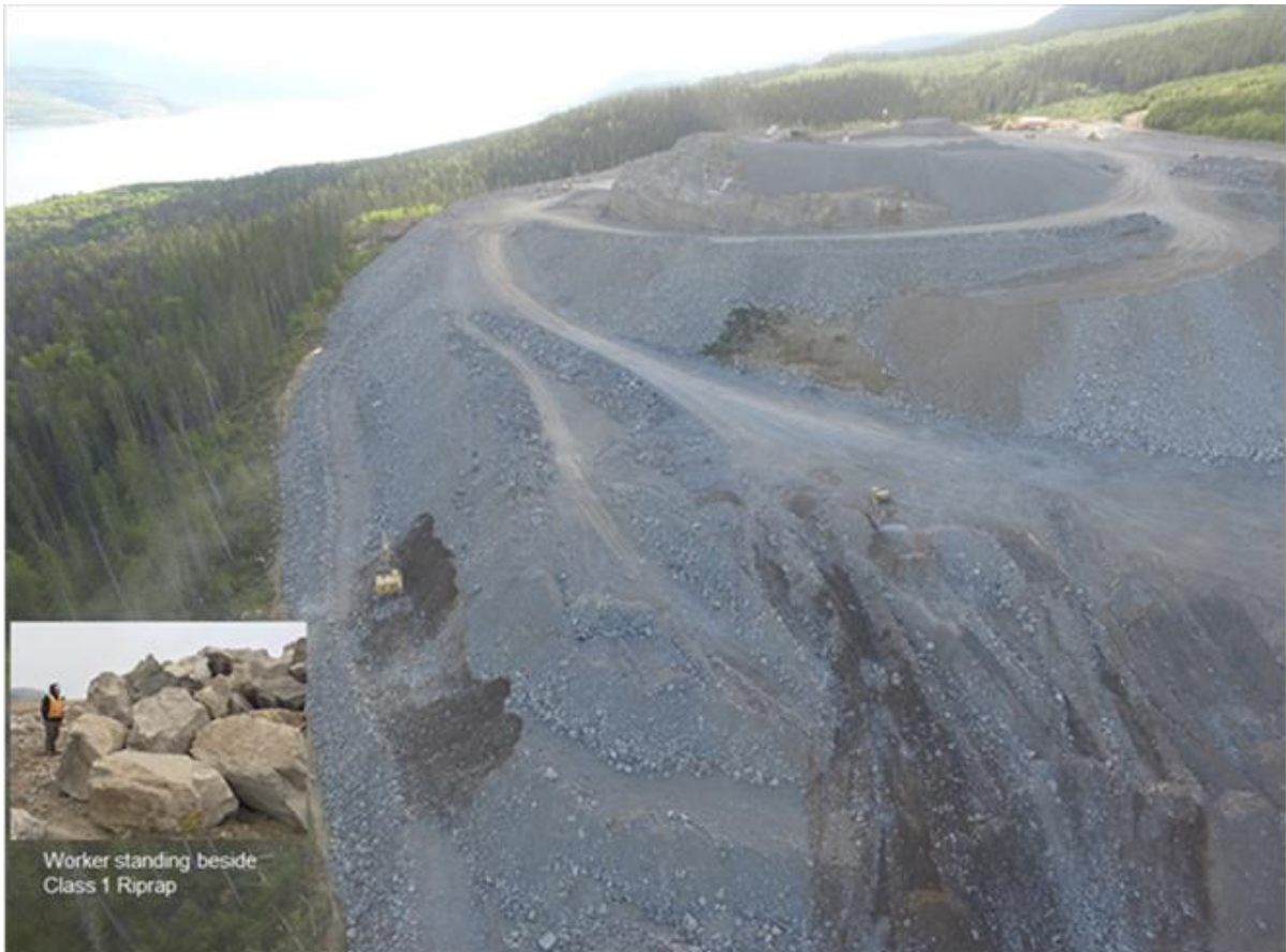
Figure 3 Sandflat Quarry at the end of Quarrying before Reclamation
