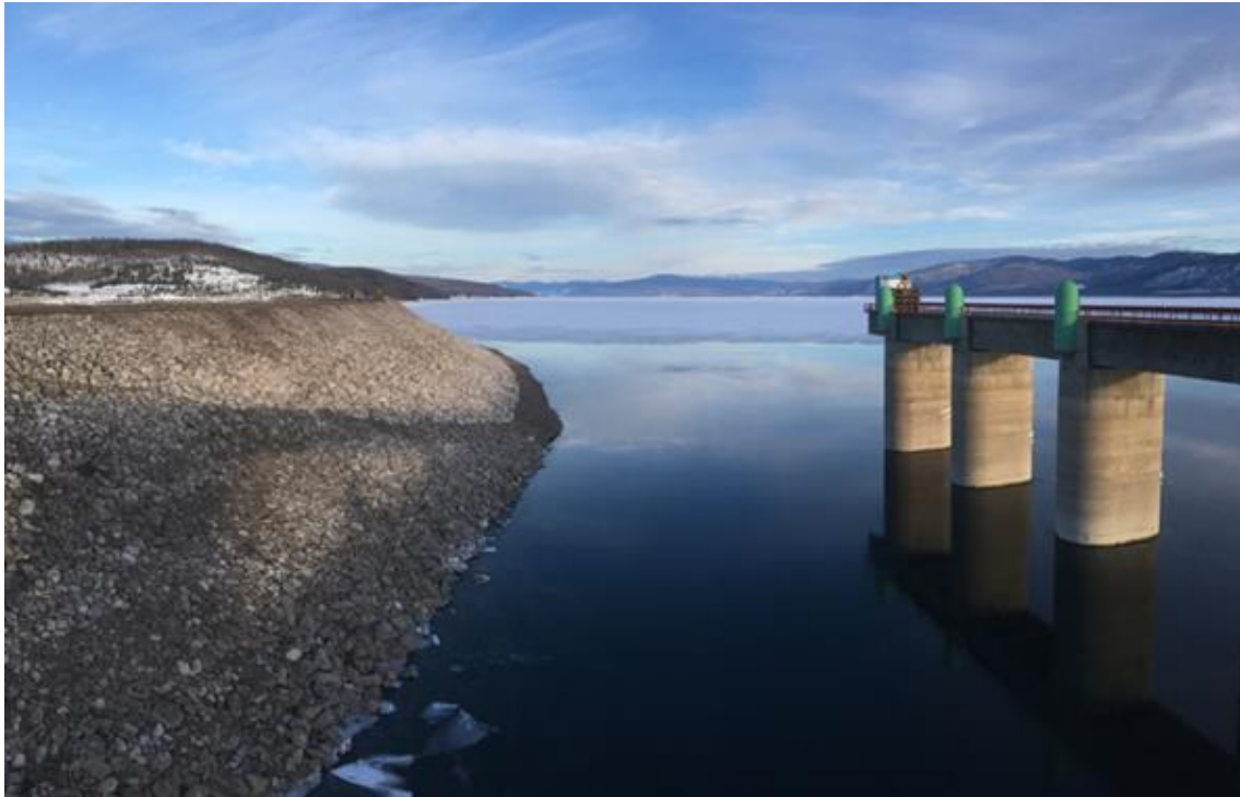
Riprap placed on the WAC Bennett Dam
