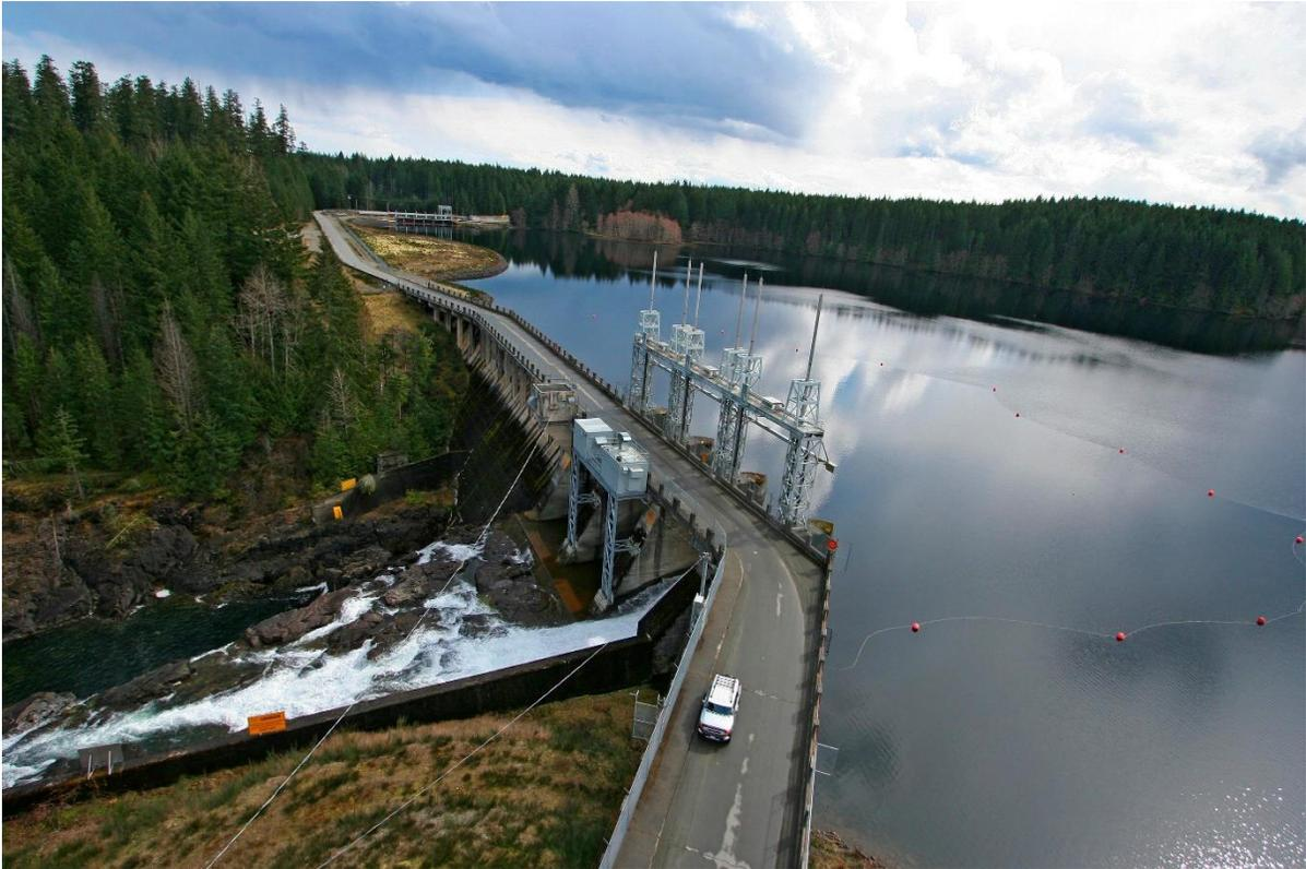
**Figure A-8 Main Concrete Dam, Spillway, new Intake and Low Level Outlets – April 2019**
