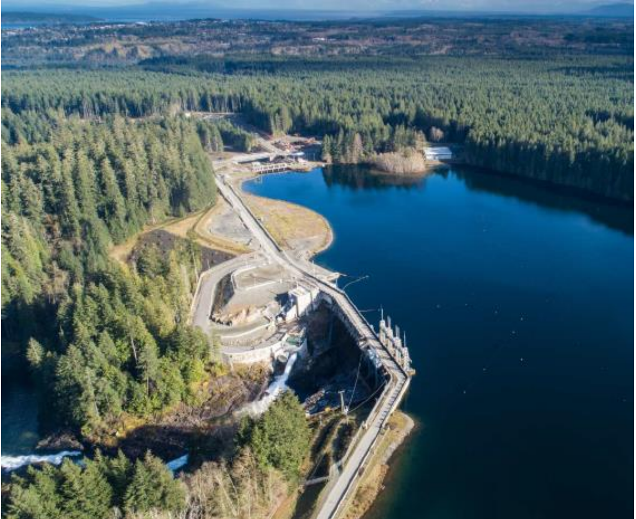
Figure A-1 Existing Dam with New Intake Structure and Water Discharging from the New Environmental Flow Release
