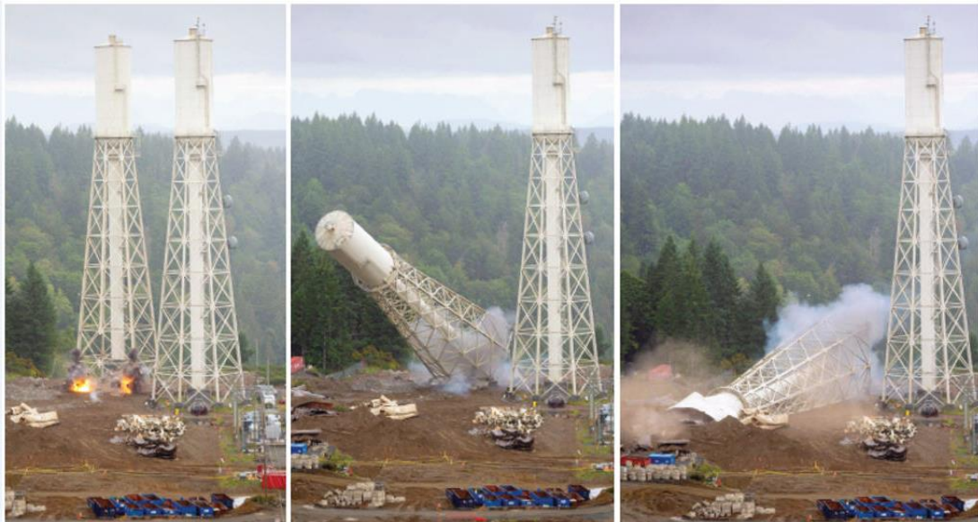
Figure A-4 2 nd Surge Tower Removal
