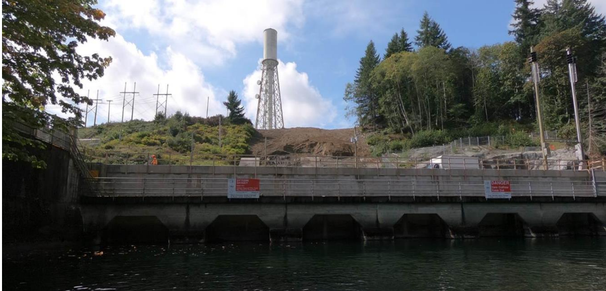
Figure A-5 Existing Powerhouse & 2 Surge Towers removed
