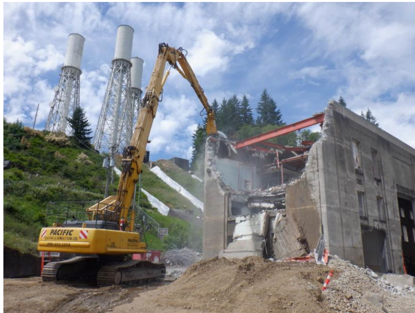
Figure A-2 Removal of the Existing Powerhouse
