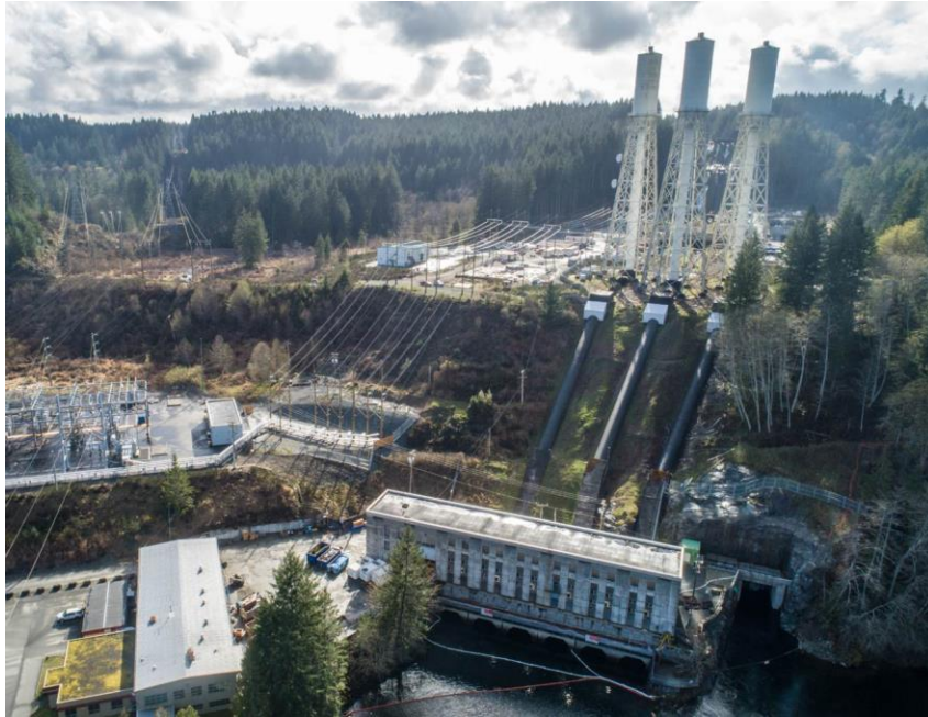
Figure A-1 Existing Powerhouse and surge towers before removal
