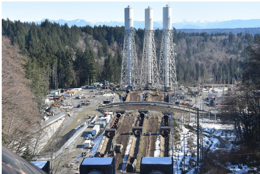
Figure A-5 View of steel penstocks removal
