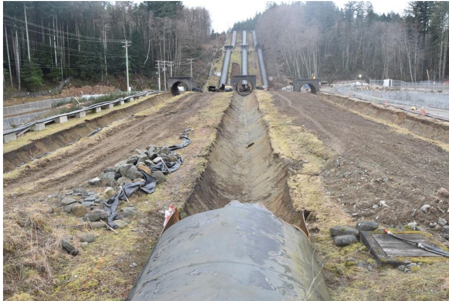
Figure A-4 Partial removal of steel penstocks
