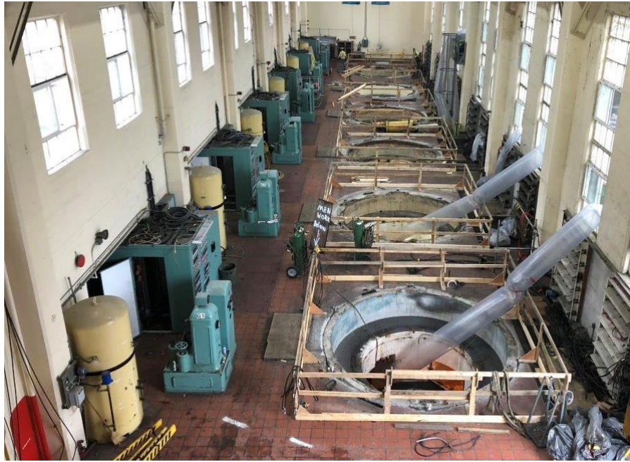
Figure A-6 Decommissioning of Old Powerhouse
