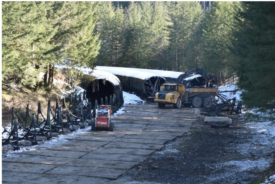
Figure A-4 Crews advancing removal of woodstave penstocks
