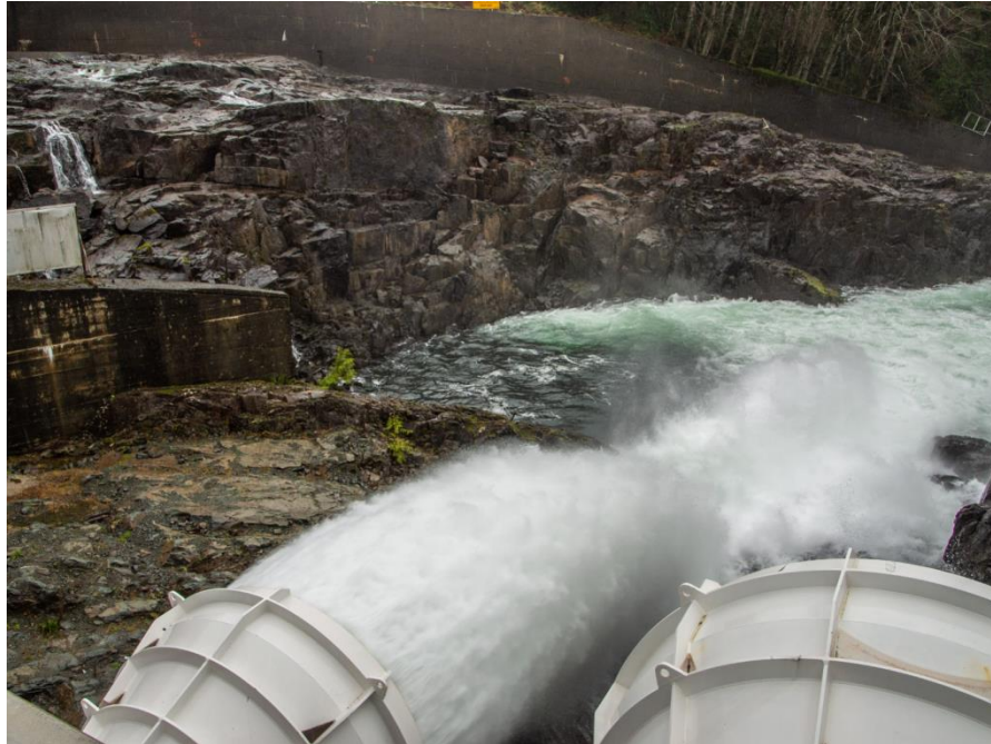
Figure A-1 John Hart water release valve passing water down Elk Falls Canyon
