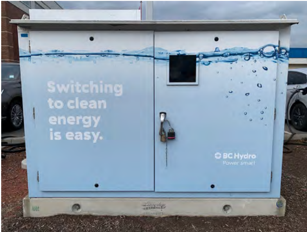
Figure 1: BC Hydro kiosk for EV charging station
