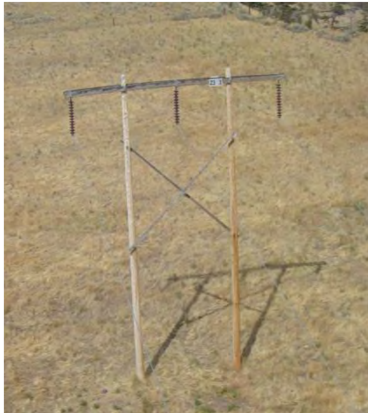
6 Figure 8-4 2L90 Circuit H-Frame Structure
