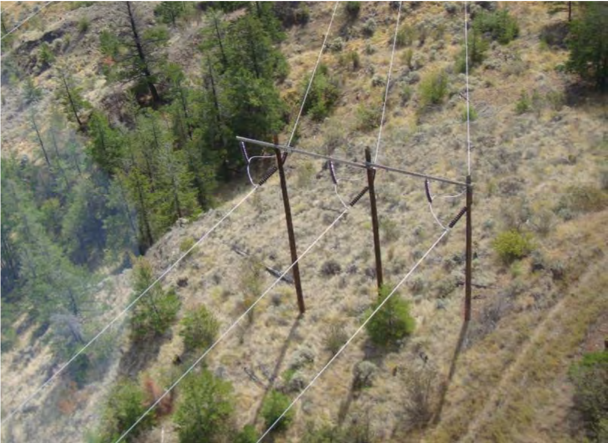
Figure 8-5 2L90 Circuit Three-Pole Structure
