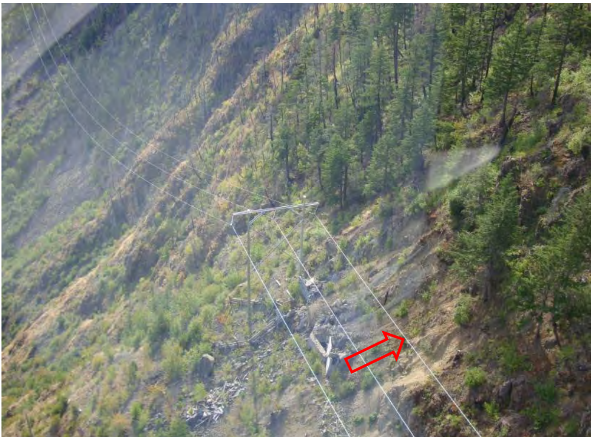
10 Figure 8-6 2L90 Span with Low Clearance
