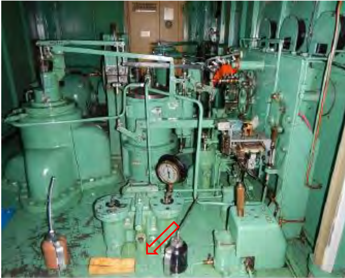
Figure 3-9 Oil Leakage from the Governors
