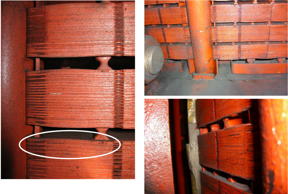
Figure 3-8 Bulging of Stator Core Laminations
