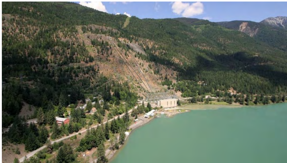
Figure 3-5 Exterior of the Bridge River 1 Generating Station and Penstocks
