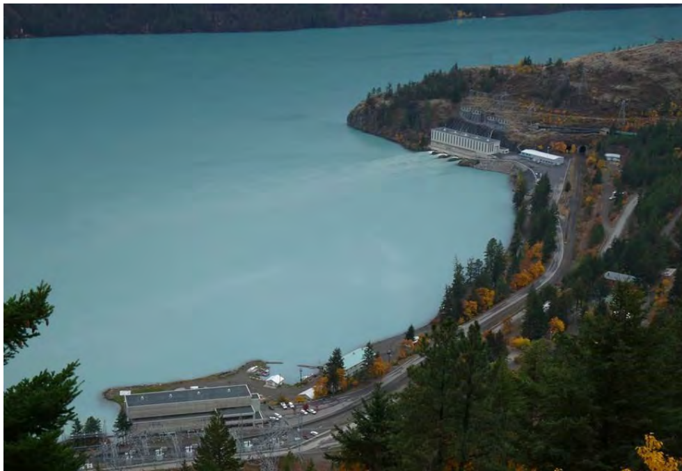
Figure 3-2 Bridge River Generating Stations and Seton Lake
