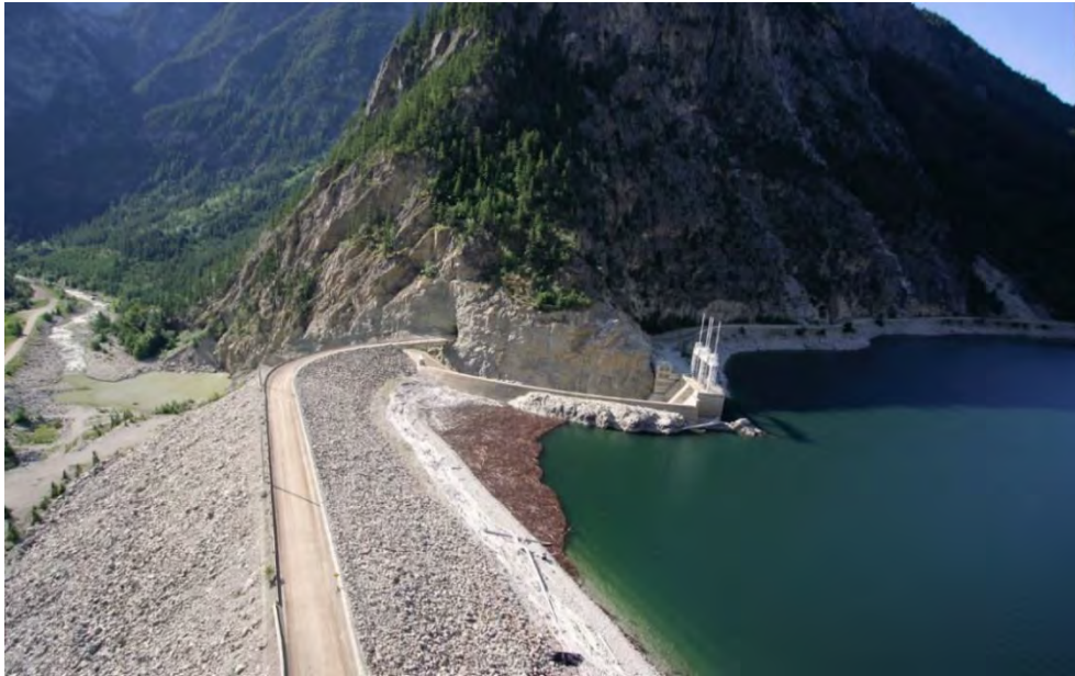
Figure 3-1 Carpenter Reservoir, Terzaghi Dam and Lower Bridge River
