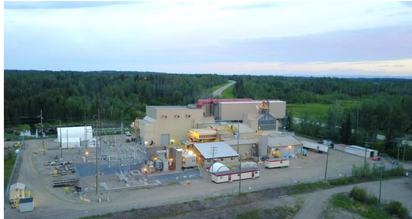
Fort Nelson Generating Station Photo credit: Ryan Sparshu
