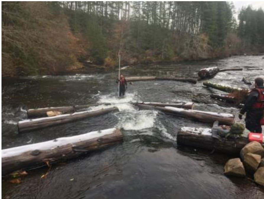
Figure 12. Looking downstream at QUN-BAR01 passage Route 7, assessed on November 7, 2017, which contains a man-made slotted fish ladder in the centre of the channel.
