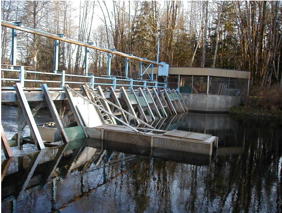
Figure 3. View downstream towards the salmon counting fence. Reproduced from Ewart and Kerr (2014).
