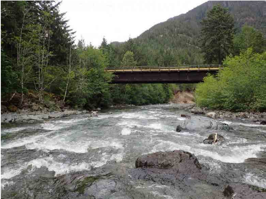
Figure 19. Looking downstream at Elk River on June 6, 2018.
