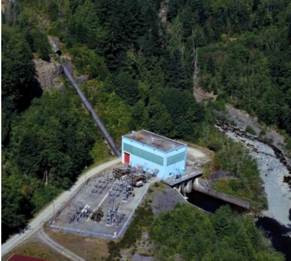
Photo 2-1 Jordan River Powerhouse
