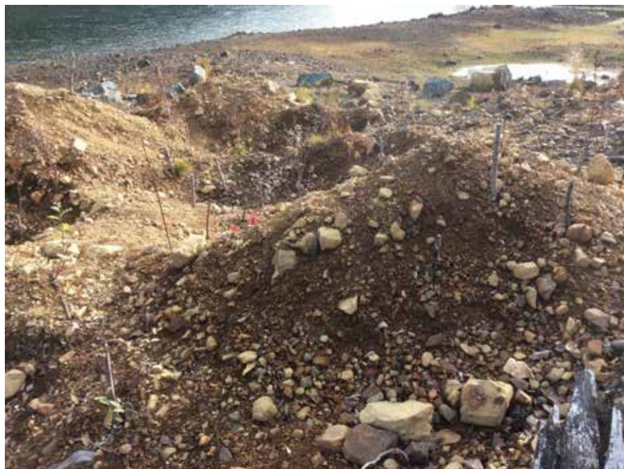
Figure 1. Machine loosened substrate in C-1ii polygon at JHT-RV02 within the islets (plot JHT-PRM29) on May 1, 2019. Hollow created for rough and loose egg carton pattern.
