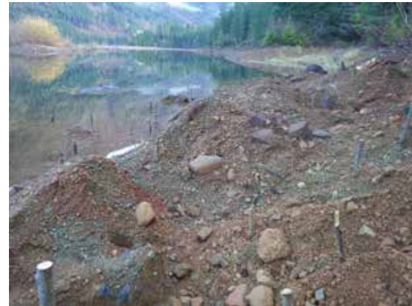
f) Looking east on 28-Nov-2018 (as-built).
